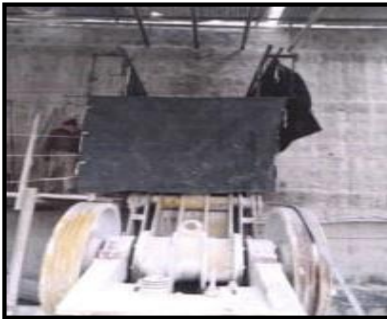
Figure-1: Covering of Primary/Jaw crusher
